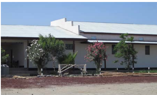
The Mille maternity hospital funded by WGP.
